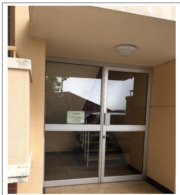
Good Natural Surveillance - But Physically Unprotected Door With Single Locking Point
