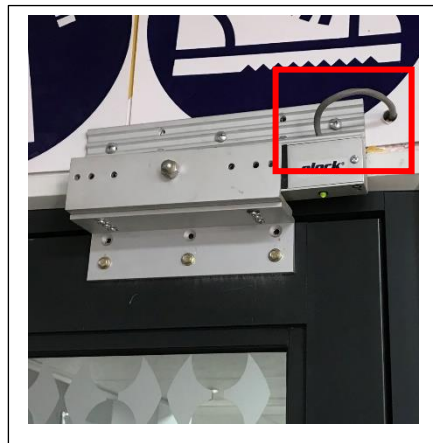
Unsafe Side Lock Wiring
